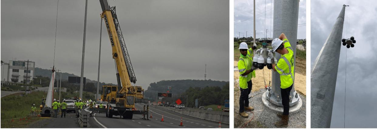
Figure 3: Validation system construction. Left: 110-foot poles are raised adjacent to the freeway; middle: Multi-camera mount holds 6 4K PTZ cameras; right: cameras are elevated to the top of the pole.
